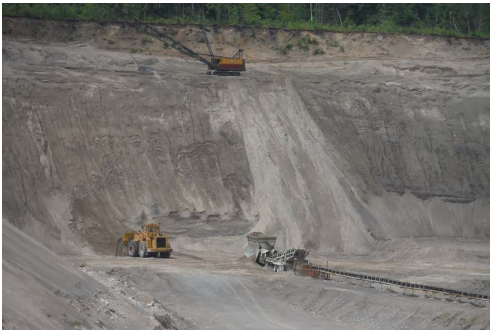
Figure 1. Vertical sand and gravel face (+/- 30m) during active extraction.
