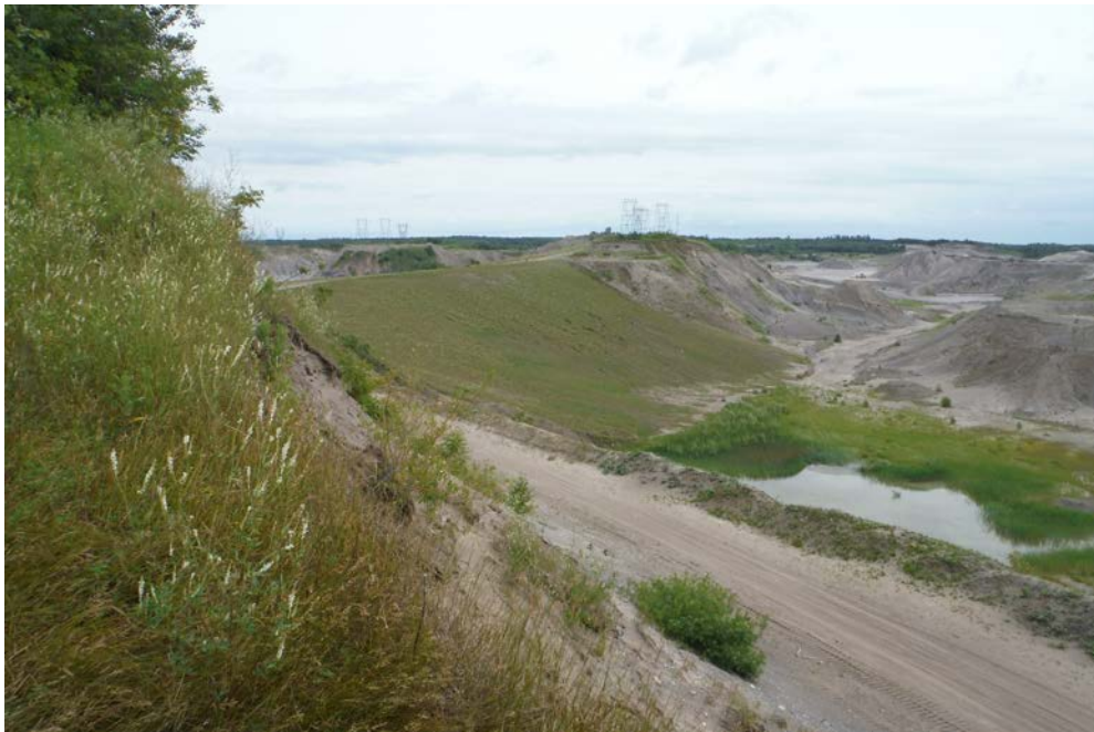
Figure 3. Rehabilitated pit face in close proximity to hydro towers.
